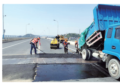
修补路面现场。郑培升/摄
