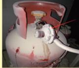
减压阀劣质、超期老化漏气
